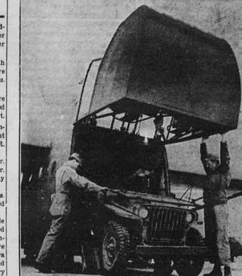
FLYING FREIGHT CAR-In carrying a jeep on a glider, the entire pilot's compartment lifts on hinges. The same procedure is
