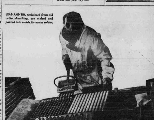
Worn-out, broken and outmoded tele- bombers . . . or be used in completely phone apparatus—even odds and ends of copper wire and lead-covered cable -are not wasted in the Bell System. Instead, at the smelting and refining plant of Bell System's Western Elec-
