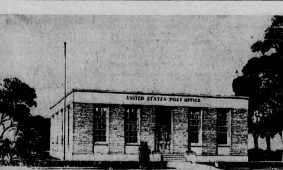
Artist's drawing shows Lowell's new $70,000 post office building, construction of which is now well under way—to be ready for use by the coming Christmas holiday season.
