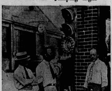
QUINCY, Mass. . . . A new traffic signal designed to stop motorists and pedestrians from "jumping the light" is shown being demonstrated by Arthur M. Loungway (right) of Endicott, N. Y., its inventor. The invention is a device consisting of an aluminum encased circle of 16 bulbs, 15 white and the 16th red. The white lights indicate the number of seconds before the light is to change, thus eliminating the possibility of being "caught" by a changing light at an intersection.
