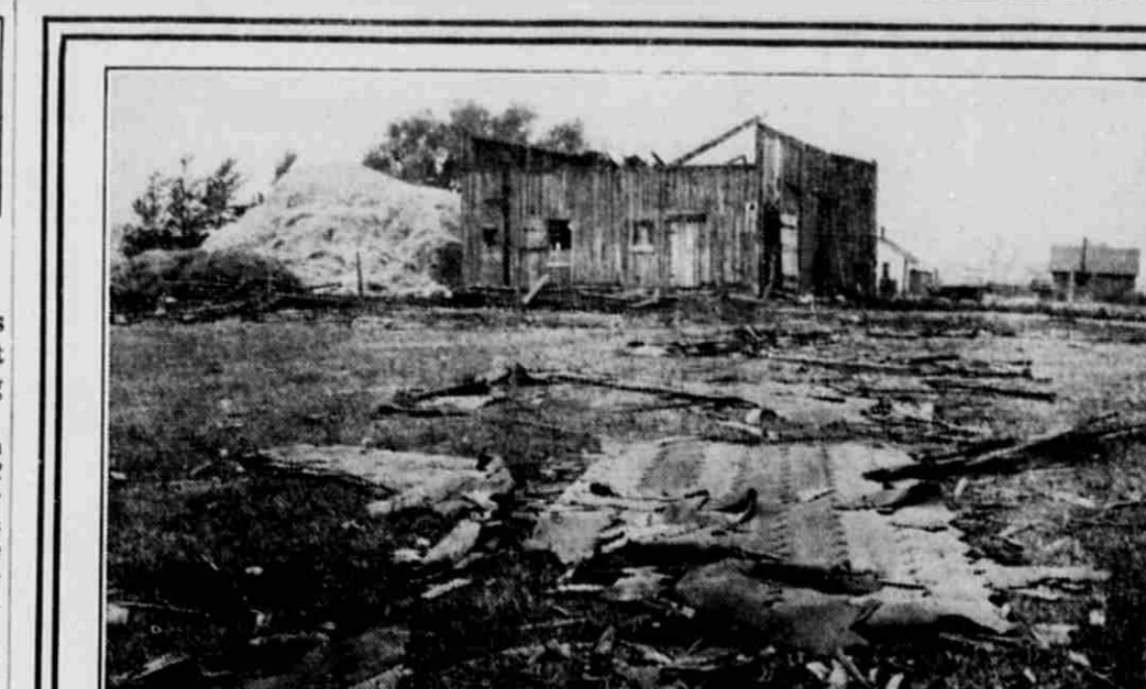
No county in Michigan is secure from windstorm loss. The above picture shows the wreck of a barn, 38 x 60, on section 3, Marlette township, Sanilac county, belonging to Lydia J. Cole. Storm July 10, 1936. This company promptly paid the loss, $10,120.
