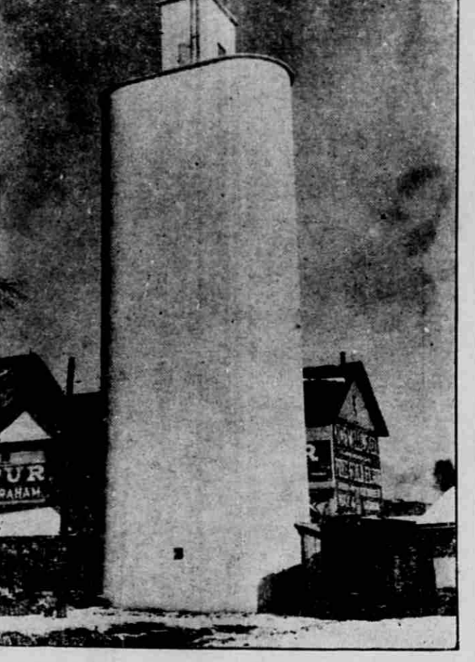
Towering 110 feet skyward, the huge granary recently completed by the King Milling Company, greets its first New Year. The huge structure is built of concrete and steel and has the capacity of more than 40,000 bushels of grain.
