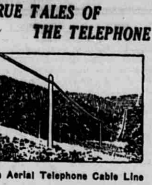
An Aerial Telephone Cable Line
