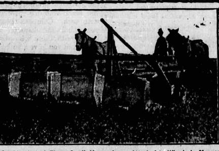
Combination of Three Small Hopperdozers Attached to Wheels in Manne to Be Pushed Instead of Pulled by Horses.
