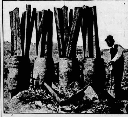
our Barrels Used With the Alternate Ones Heated by Means of Fire Beneath the Extended Ends of the Pipe.
