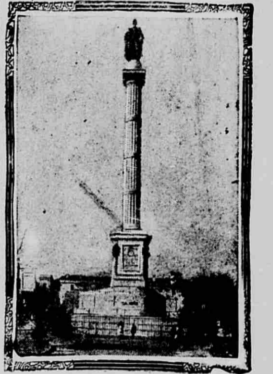
CALHOUN MONUMENT, CHARLESTON, S. C. covered with red ones. We went into St. Michael's church, one of the oldest churches in the South, twice injured by fire, and the walls cracked during the great earthquake. The three walls are lined with memorial tablets; the pews are of the old style, high ones,
