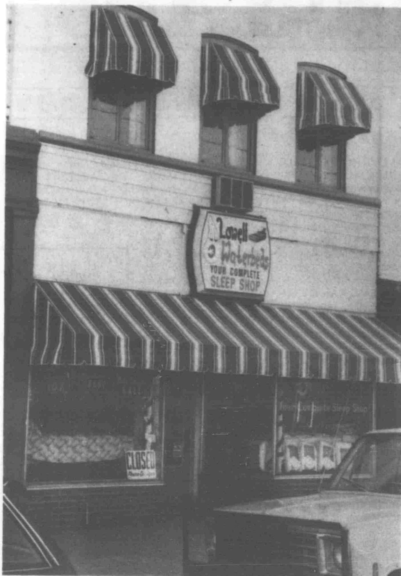
The front of Lowell Waterbeds was adorned with new awnings on Monday, adding them to the ever growing list of Main St. businesses that have spruced up their buildings with the aid of Community Development Fund money. The building is owned by Tom and Pat Covell who reside in the upstairs apartment and lease the main floor to Lowell Waterbeds. Our Main Street looks a little nicer as each of these awnings goes up.
