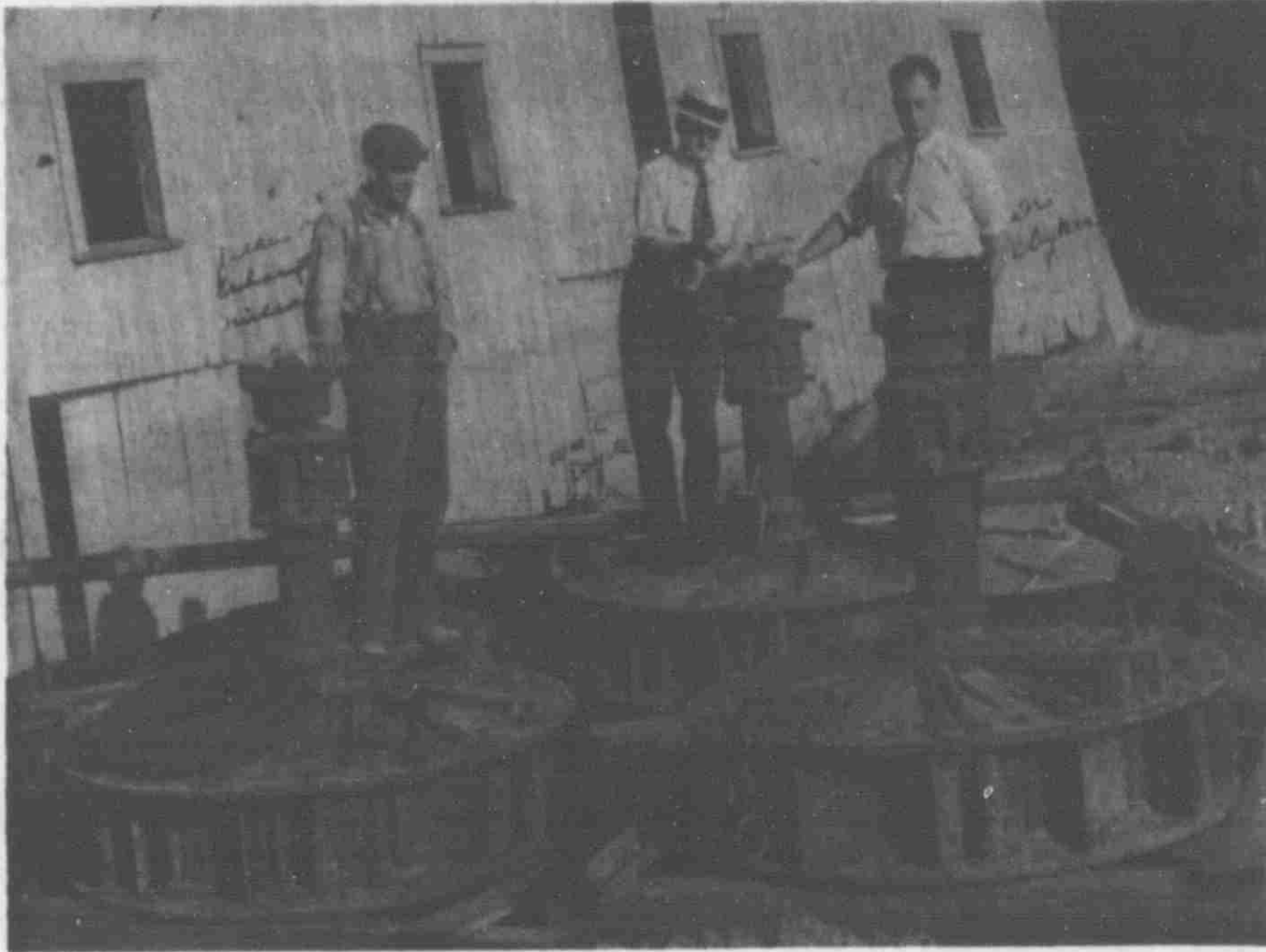
Pictured above are the milling turbines that are now on display on Main Street. This picture was taken in 1937 when the mills on both sides of the Flat River suffered washouts. The new concrete dam and races were installed at the same time.
