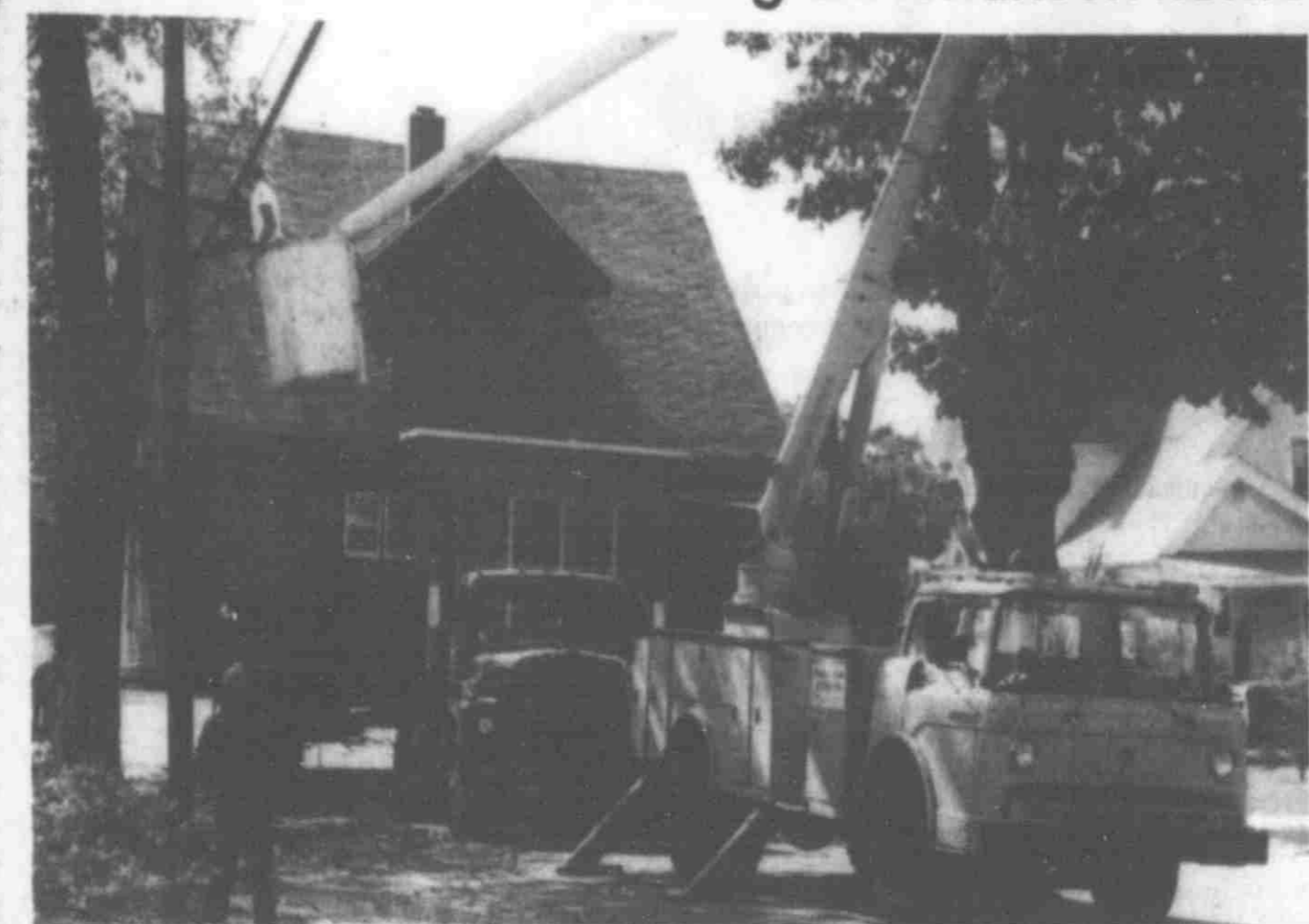
The old Christiansen Home made its move up Jefferson Street last Tuesday. There were a few tight squeezes along the way, and many limbs had to be trimmed. Work has already begun on the First United Methodist Church parking lot that will be built on the home's old site at the northeast corner of Jackson and Main.
