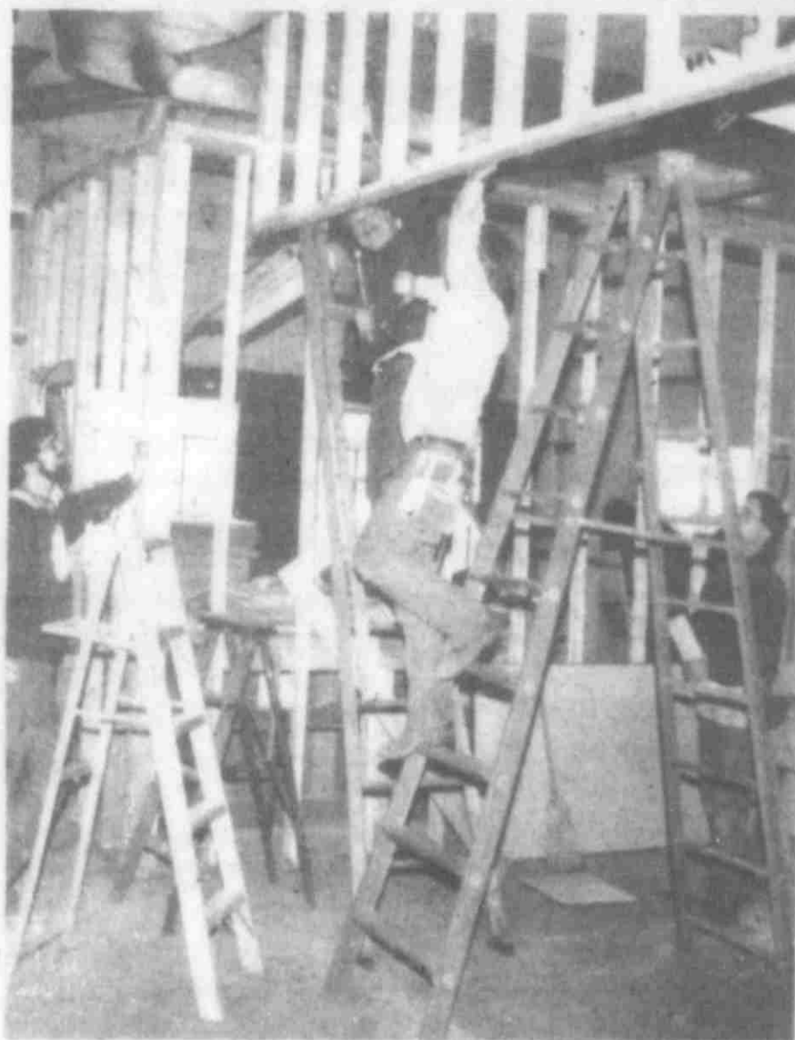
Lowell Area Arts Council volunteers work to erect a partition in the new LAAC headquarters.
