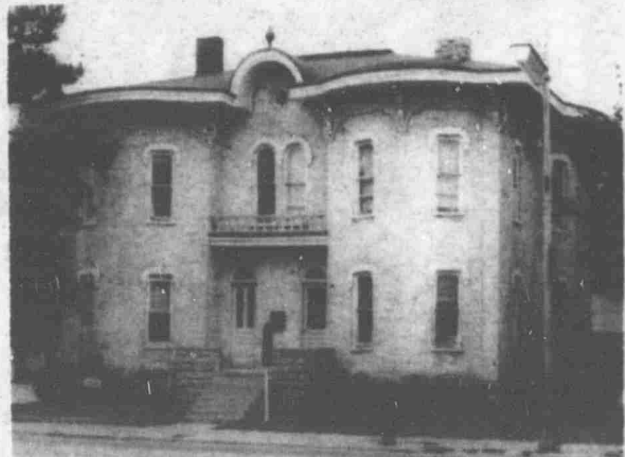
The Lowell Library has been the recipient of extensive outside renovation thanks to the Look Memorial Fund.
