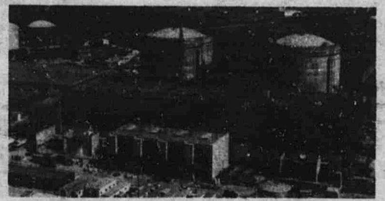
The Midland Nuclear Plant in the home stretch of construction.
