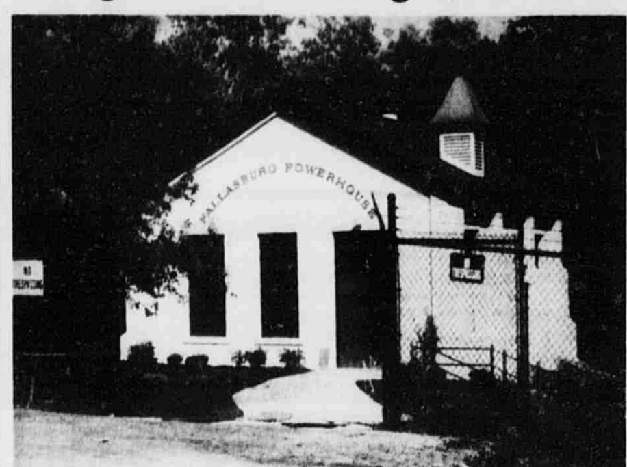
This view of the "Fallasburg Powerhouse" typifies the extensive renovation that has transformed both the powerhouse and dam into working facilities rather than white elephants or dinosaurs.
