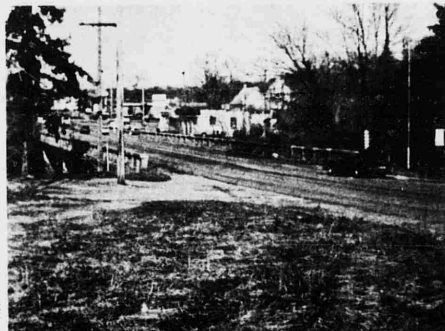
This bridge over the Thornapple River in the Village of Cascade will be replaced by a new one this year. Businesses can be seen in the far background. This picture was taken last November.
