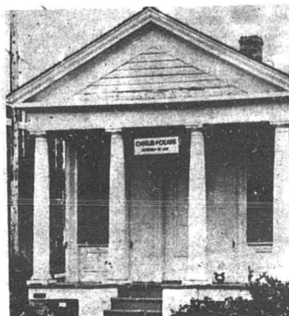
The Calkins Law Office of the Grand Rapids Public Museum is now opened each Sunday afternoon, 2:30 to 4:30, through September. This completely restored 1836 Classic Revival frame building, is located adjacent to the Public Museum in Lincoln Place Park in Grand Rapids. Admission is free.
