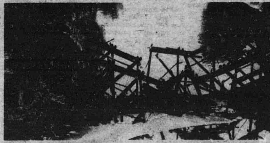
The Ada Covered Bridge went down in flames on Sunday, September 9, 1979, about 9:40 p.m. It had only recently been restored after the roof collapsed under the weight of snow and ice in February of that year. Investigation of the suspected arson is still open. The 125-foot bridge was a Michigan historic site, built around 1867 by Will Holmes and Jared Braze on the same patent as Fallsburg Bridge and White's Bridge.
