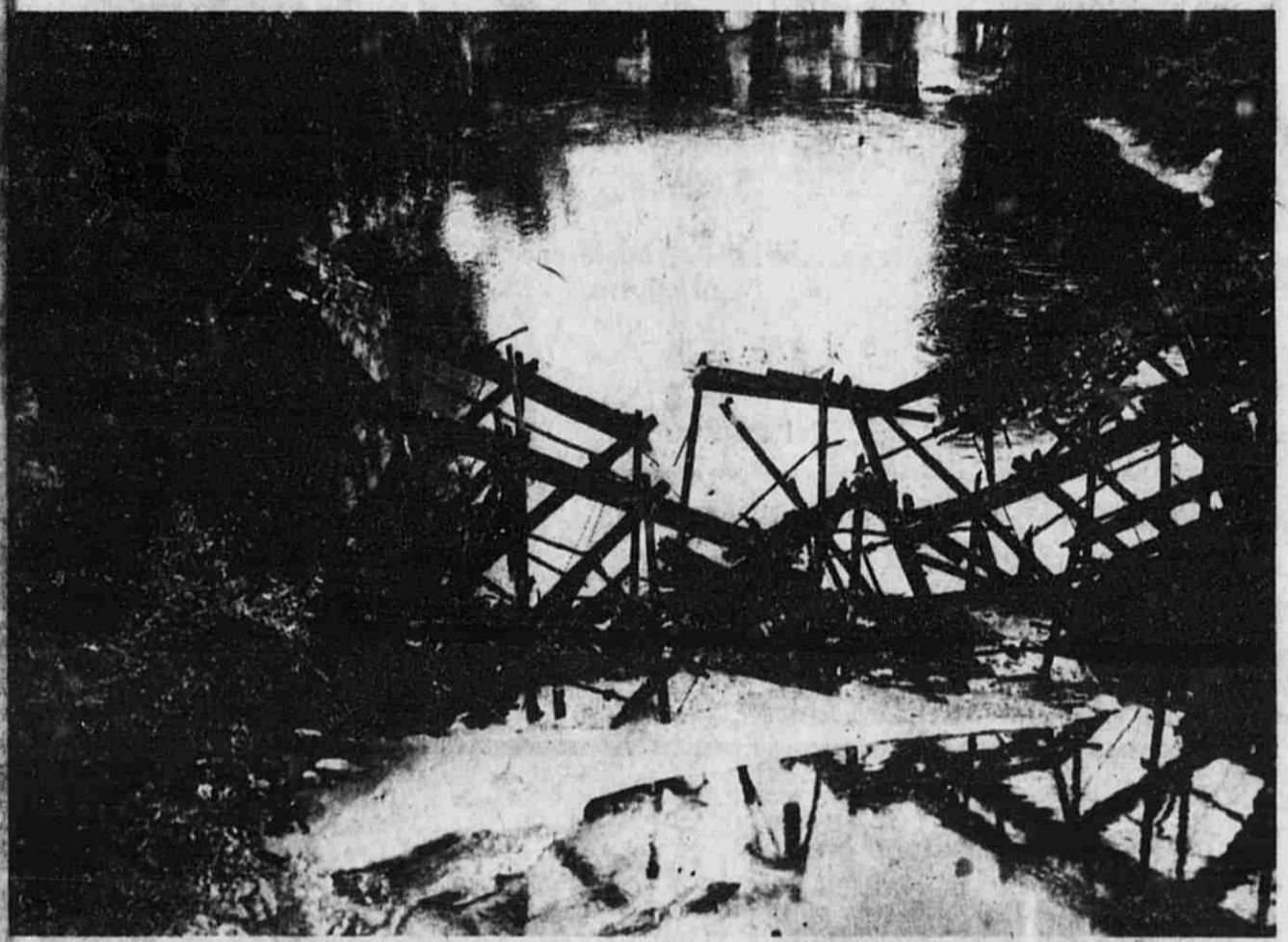
The Ada Covered Bridge went down in flames last Sunday night about 9:40 p.m. Eight area fire units responded in minutes but the structure was nearly engulfed when they arrived. The roof and sides were completely consumed and the end nearest the ball diamond at Fase Park fell into the river. There were no plans to rebuild at press time.
