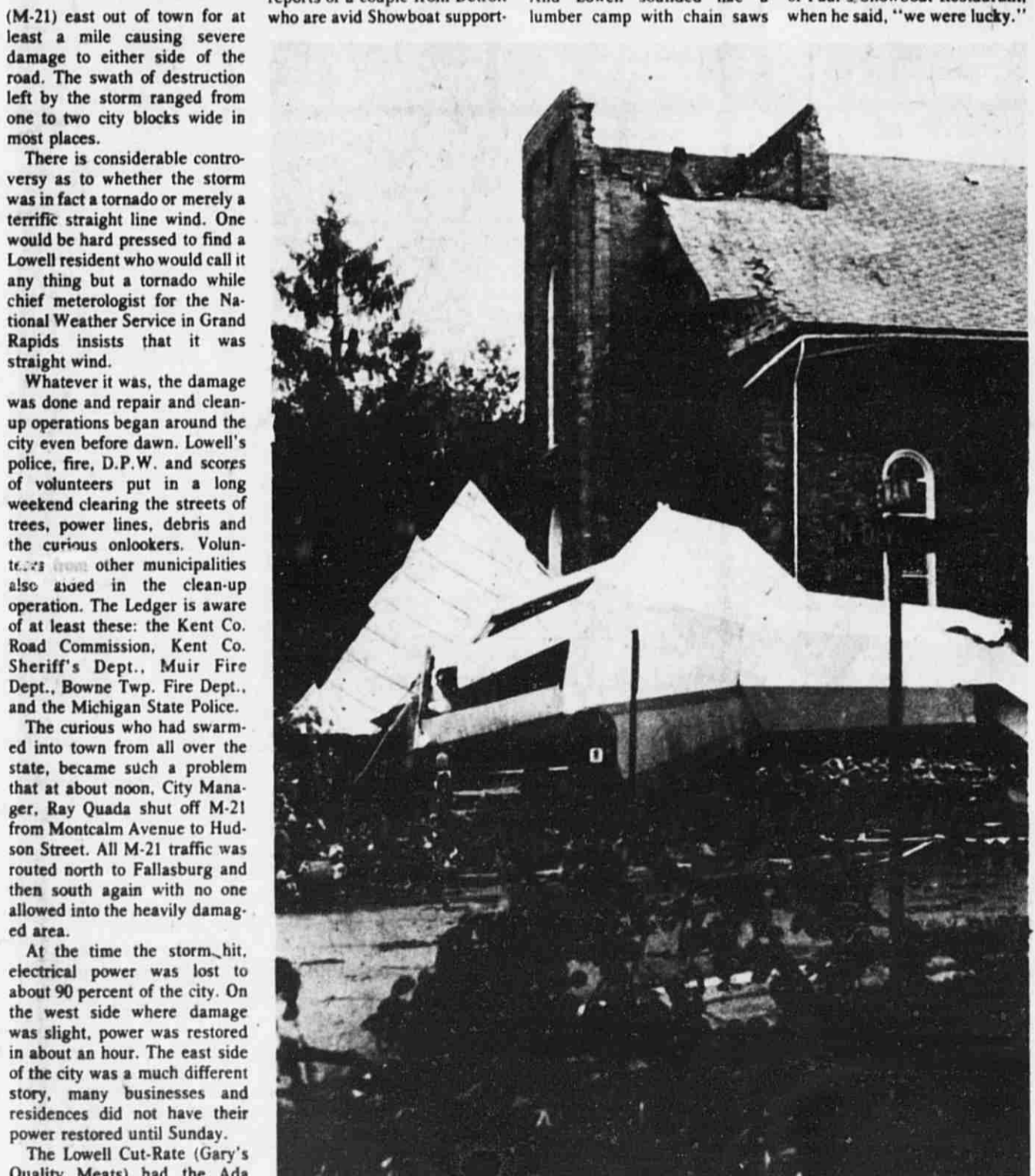
Ripping the steeple off from the First United Methodist Church of Lowell was one of the most sensational bits of destruction that the wind dealt out. The belfry portion of the steeple is more than 100 years old, but the very top section of the structure was erected in 1967.
