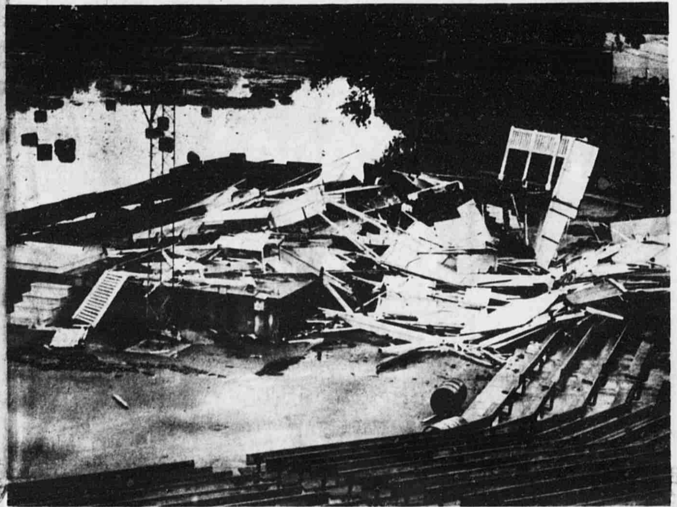
The Lowell Showboat which less than a month ago was steaming around Cattail Bend in all her glory, was reduced to the above pictured mass of rubble by the windstorm. The light towers at either end of the stage incredibly escaped being damaged and must have been missed only by inches when the debris from the Showboat was hurled past. A volunteer work day is scheduled for Saturday, August 26, to clean up the mess.
