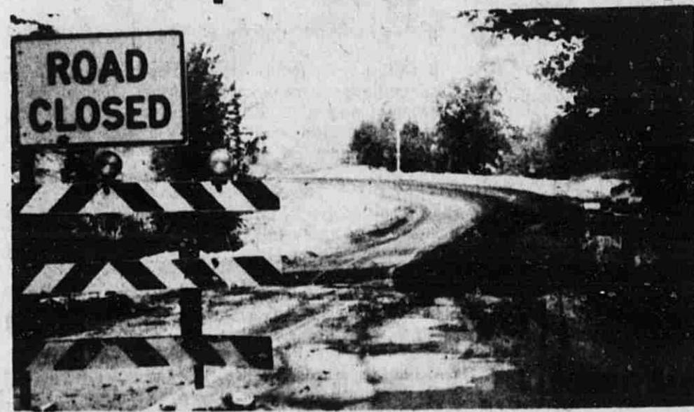
Relocated Forest Hill Avenue is about ready for blacktopping.
