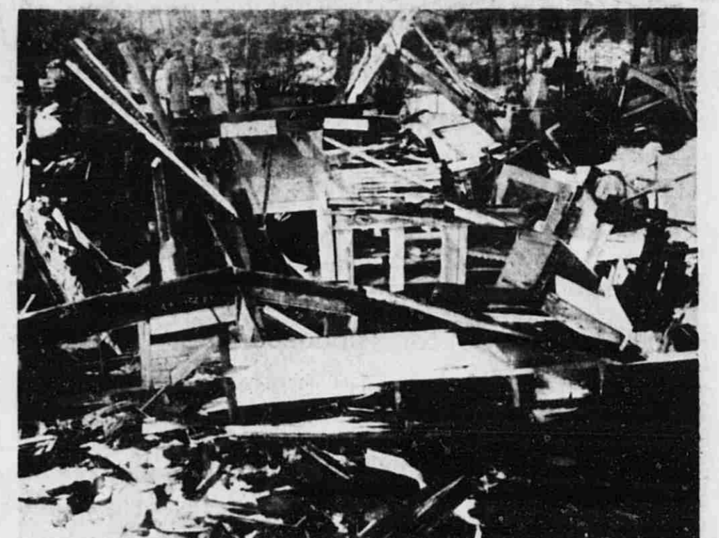
A home owned by Ronald Richards at 706 High St., Lowell was completely destroyed recently when it fell into the hole that was to be its new basement. The Ledger was unable to contact anyone who knew anything about the accident but the house had apparently been jacked up and a new basement was being dug under it when the house went down.
