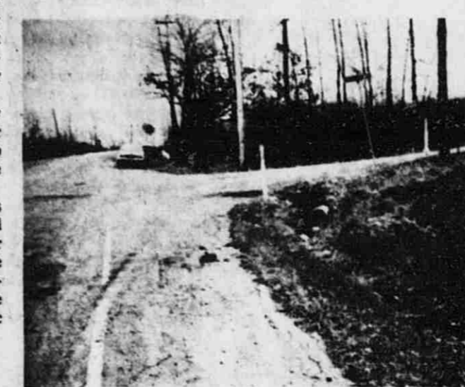
Michigan Street NE, at left, will start angling to the right, cross Greenwich Avenue, above right, and continue southeasterly to the new East Beltline. This relocation will eliminate the blind corner, right photo, caused by the "solid" railing of the East Beltline overpass over railroad tracks. A new five-lane overpass will replace the present one.
