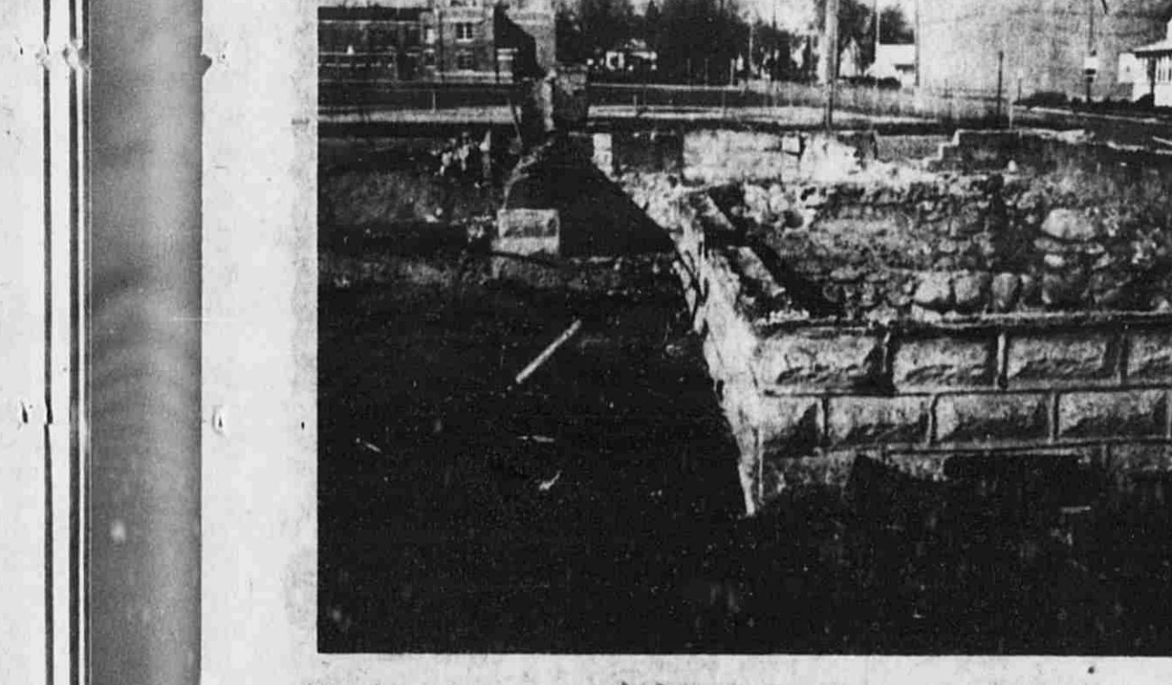
Makes Way For Parking Lot "You may have noticed that the city owned two story home on the corner of Monroe and Avery Streets, has been torn down. In the above photo, all that remains is the foundation. The property was purchased by the City to create more parking for the business district. City Manager Ray Qanda says that the area should be ready for use within two weeks. The lot will be paved sometime next year."
