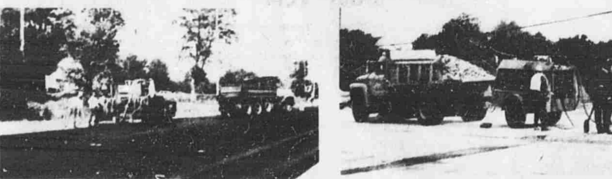
Resurfacing of Cascade Road between Int. 96 and Hall St., SE, is taking place without through traffic having to be detoured. Backtracking near Int. 96, left photo was done first. A truckload of asphalt is being backed to the spreader, above center, where workmen help smooth the asphalt and operate the spreader. A roller, now shown, compresses and "hardens" the backtracking.
