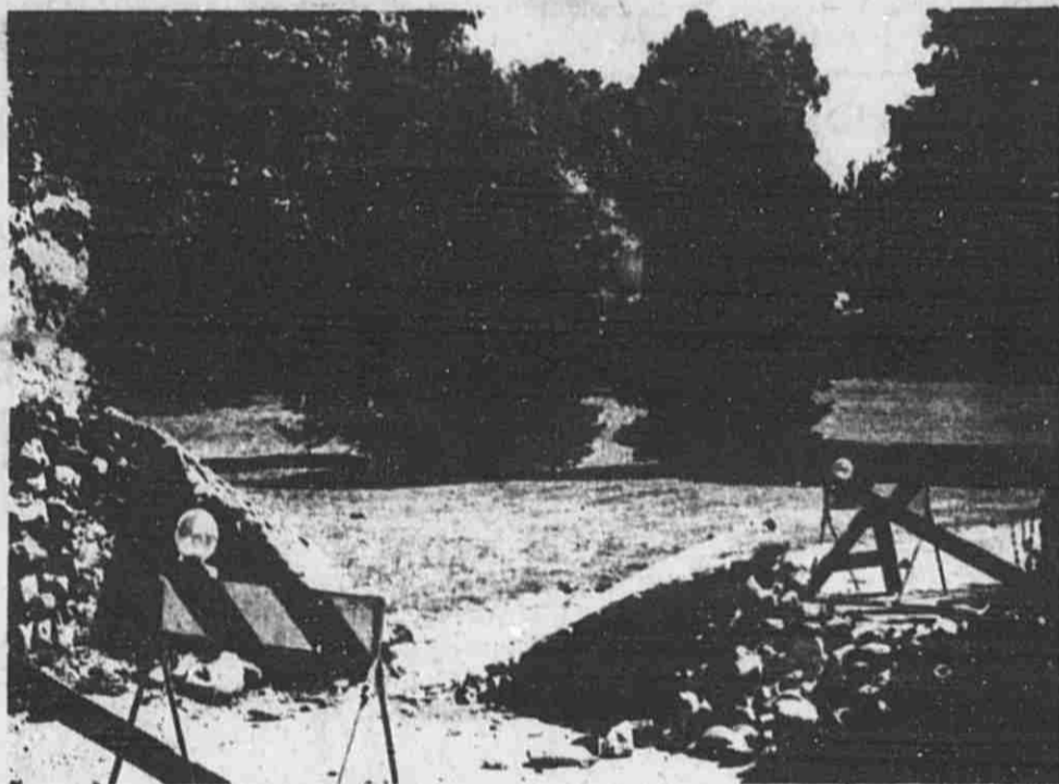
Above, what is left of the historic "Falls Arch" at Fallsburg Park. The arch, erected in 1930, was completely demolished when the auto in the top photo impacted with it at an apparent high rate of speed.
