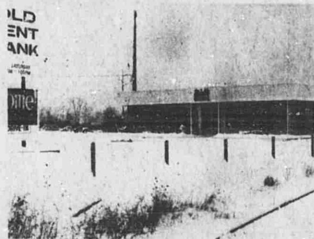
Old Kent Bank opened their new Ada Branch Office Thursday, December 18. The new Ada branch is now the farthest east of Grand Rapids of any of their over thirty offices. The office is located on Highway M-21 just west of the Amway Plaza.
