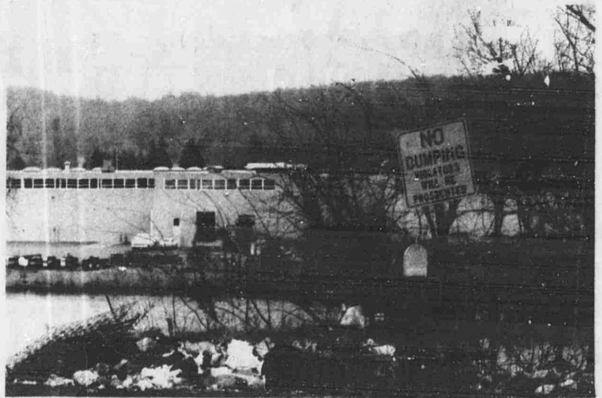
Trash stown along the bank of Flat River north and just outside the City limits in Vergennes Township. The sign is apparently no deterrent.
