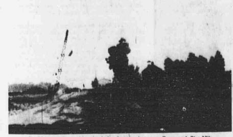
Looking north on Lincoln Lake Avenue between Four and Five-Mile Roads are two huge piles of muck, right, removed to make way for sand and other proper fill prior to the rebuilding of this part of the county road. A crane, left, removes unwanted earth from the right-of-way and dumps it far from the road, part of which had already been taken away, center background.
