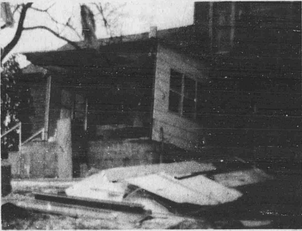
This 36th Street home south of Lowell received heavy damage.
