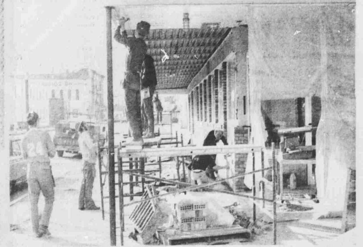
Workers put the finishing touches on Lippert's new building at 413 East Main Street, and they strive to make the completion date of February 1, when the new store will be opened to its first customers.
