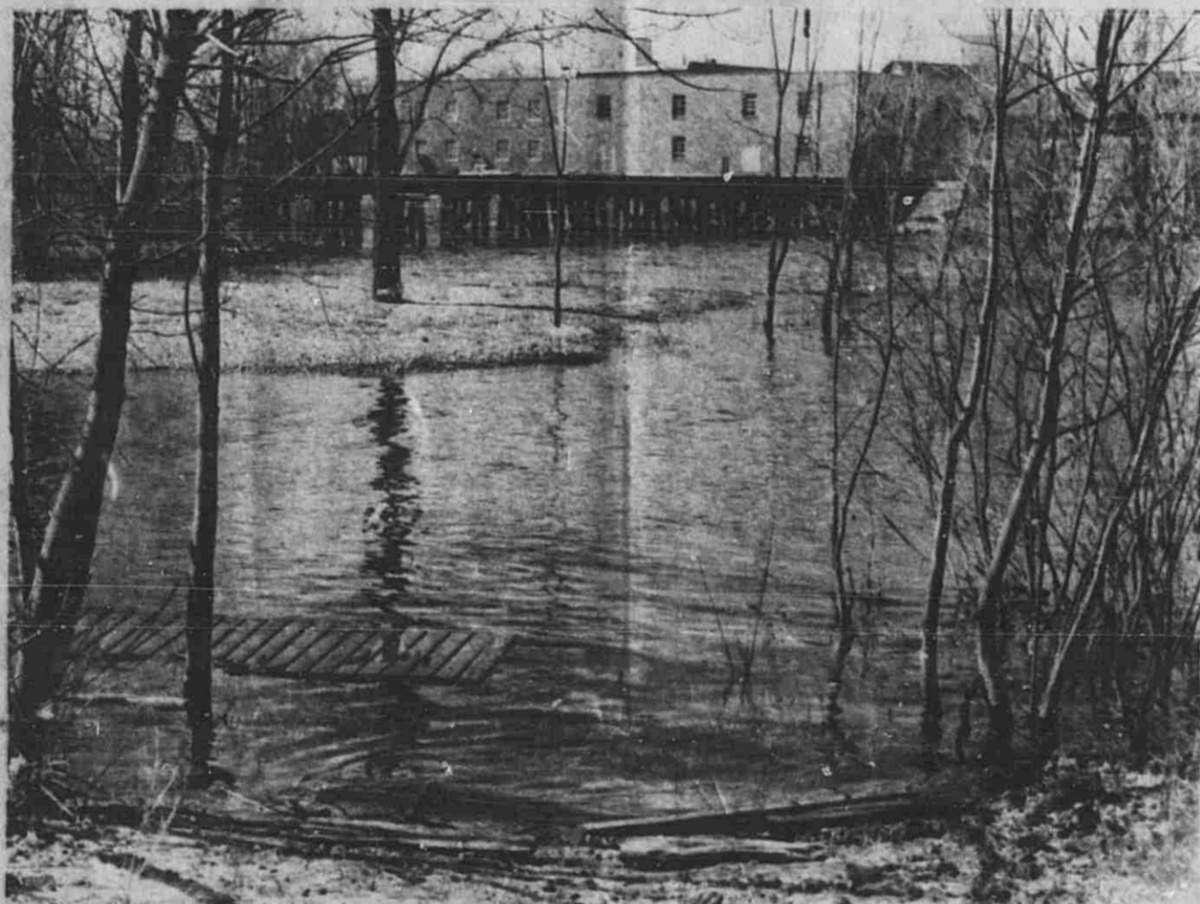
SPRING FLOODS - Made of melting snow and occasional rainfall have done their damage to Lowell's Island Park, washing out the bridge and nearly covering the island. The waters are now receding and thus far there have been no reports of damage to other homes or property in the area.
