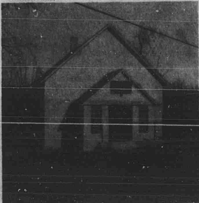
A fresh coat of paint has been put on the new Lowell Community Center, 10763 Grand River Drive.
