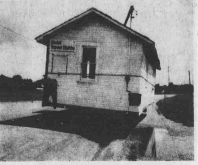
A pair of men's red flannel underwear was used as a warning signal to following motorists that the familiar building on the corner of 28th Street and Cascade Road, adjacent to Slater's Mobil Station was moving to a new home.
