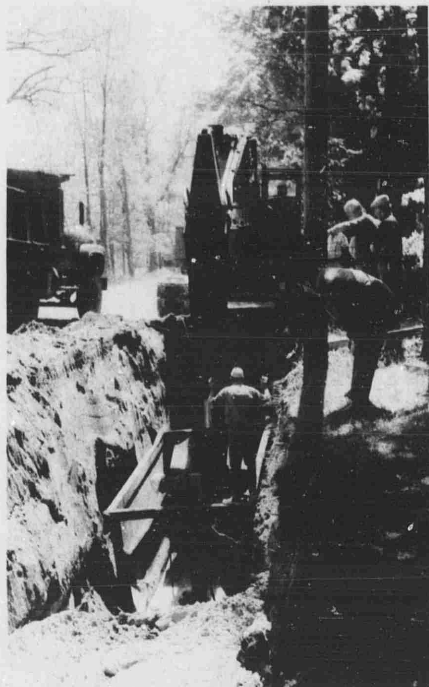
ON THE MOVE — Two major construction projects in the area are beginning to take shape. At the left, workmen are shown as they continue installation of a new sewage line in Cascade Township along the Thornapple River Drive . . . which has caused constant tie-ups in local traffic. Above is the new Schneider Village, a housing project for senior citizens, as it appeared this week in Lowell. A fall completion is expected.
