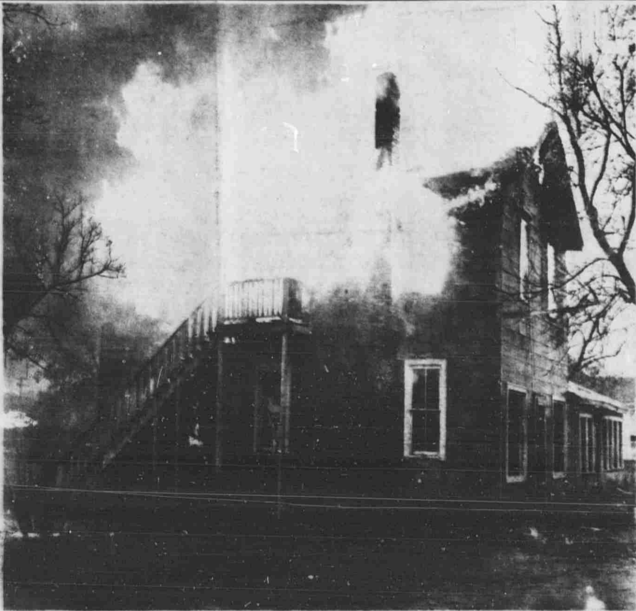
NO FEAR HERE - There were no occupants, no furniture... even no windows for firemen to break when this house caught fire in Lowell. It was owned by the city and intentionally razed... thus giving firemen an opportunity to practice fire-fighting techniques.
