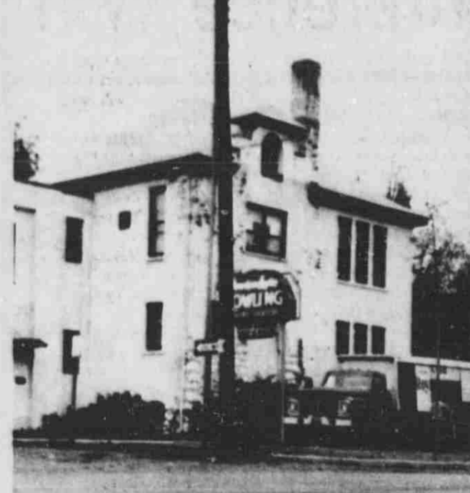
FORMER SCHOOL - Few residents who pass this building every day realize that the old East Ward School in Lowell is now the site of the American Legion Hall and bowling alley. . . but the outline of the school is very much in evidence.
