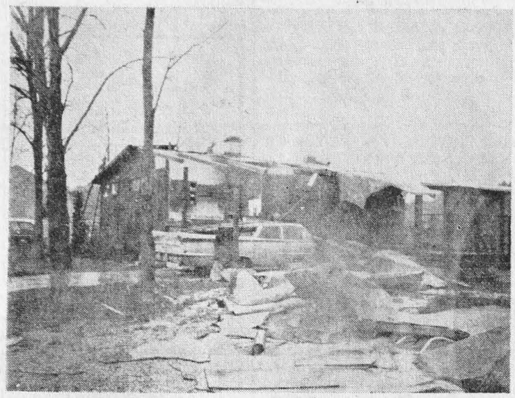
The second tornado caught the home of Mr. and Mrs. Fred-eric Ross of Thorncrest Drive and tore it to pieces. This was one of seven homes completely wrecked. Help was quick to arrive. 23 Cascade firemen reported for duty, along with others who volunteered.
