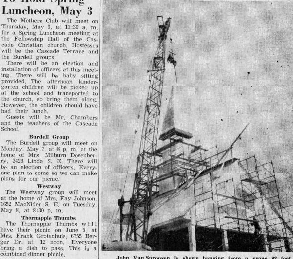
John Van Spronsen is shown hanging from a crane 82 feet in the air, on a 6-ft. cross which was placed on the steeple at the Cascade Christian Reformed Church at 6631 Cascade Rd., S. E., last Wednesday. Just before this picture was taken, the steeple was set into place and the cross was the finishing touch, which nearly completes the new sanctuary, that was started last October.
