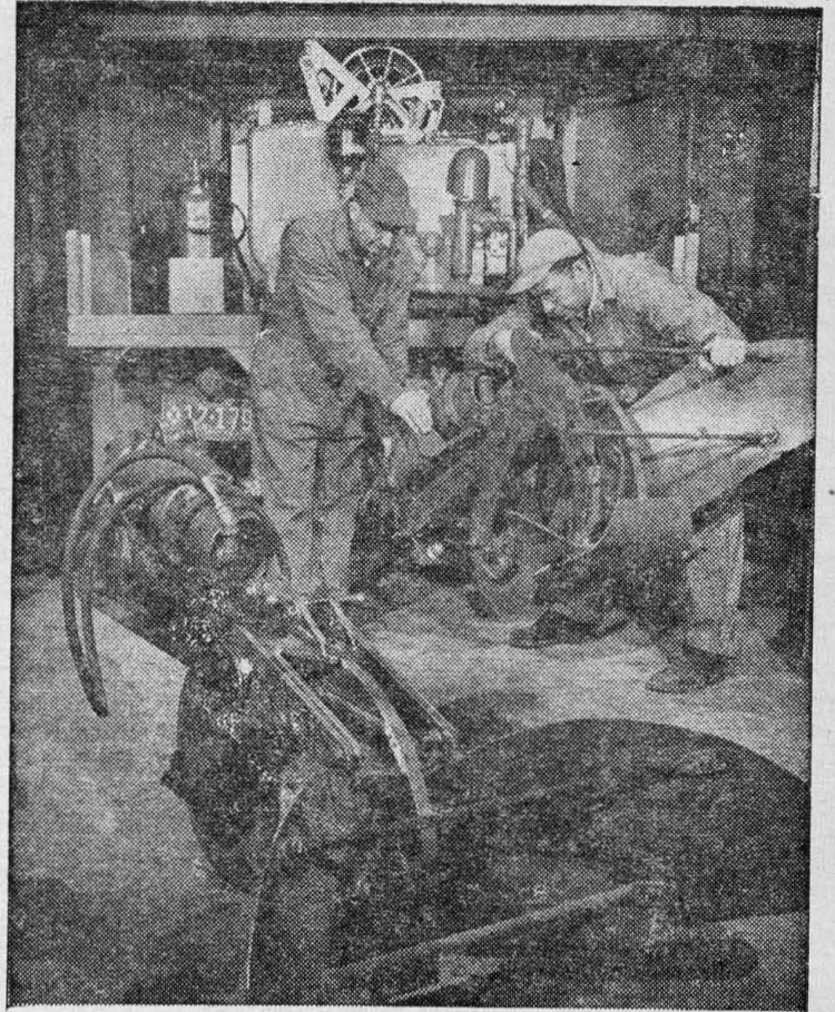
Machinists make final adjustments to a firelane plow assembly at the Conservation Department's forest fire experiment station as the spring-time threat of forest fires approaches. During the winter, crewmen at the station keep busy repairing and improving mechanized equipment to aid fire fighters in holding fire damage losses to a minimum.
