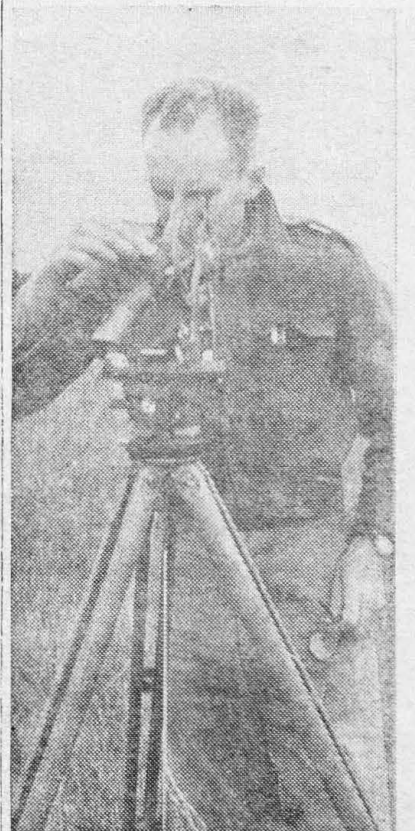
John Loucks, surveyor with J. G. Daverman Company, architects and engineers for Forest Hills High School new construction, is shown here laying out the buildings on the Hall Street site. The surveying crew has been busy laying out the four buildings, drains, water mains, and streets of the new high school that will house over five hundred students in just a few years.
