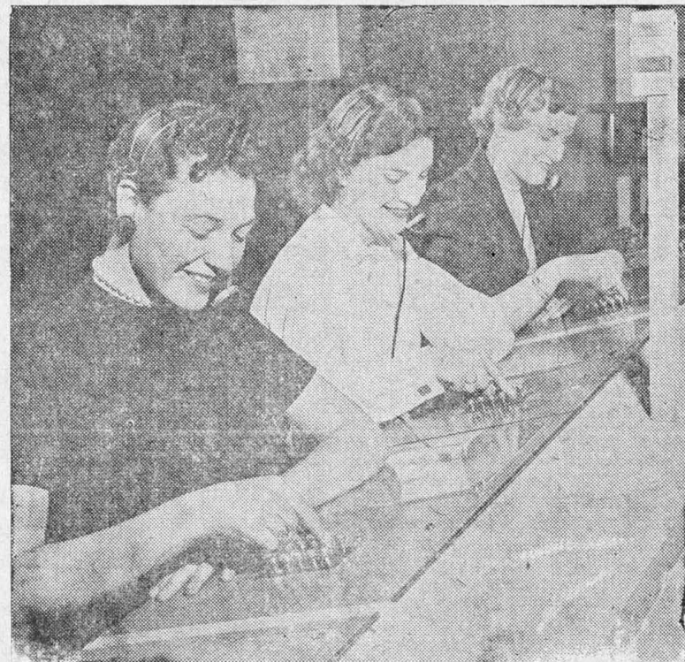
Telephone operators at Grand Rapids Centralized Automatic Message Accounting center will ask callers for the number of the phone they're calling from, then register the number at special keyboards. This information is transmitted to automatic message accounting machinery.
